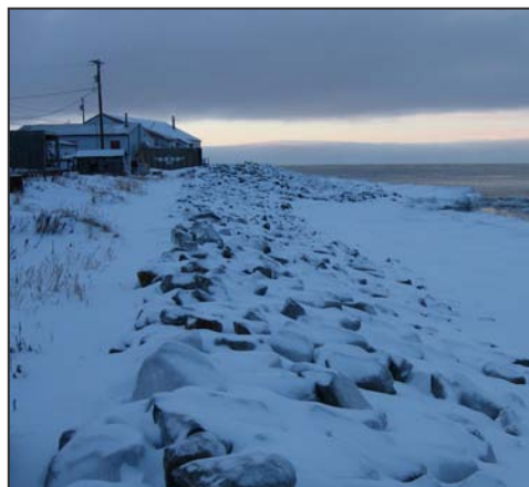
Boulders along the beachfront at Shishmaref, AK, are meant to protect the coastline from further erosion.
